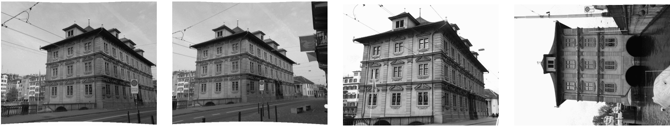
Figure 8: Four views of one side of the Zurich City hall which are used in the plane sweep to determine the window indentations.
